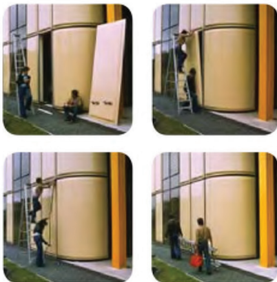
Herman Miller factory cladding system https://www.hermanmiller.com/en_gb/stories/why-magazine/the-bath-brief/
