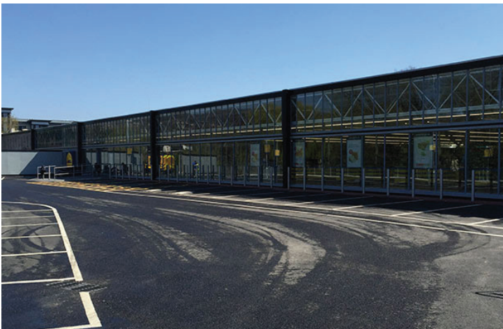
Cabinet Makers, now commercial units. Sir N. Grimshaw, 1967
